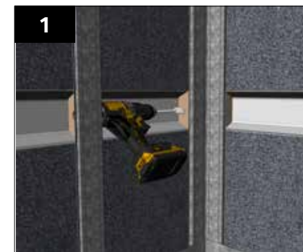
Using a hole saw or spade bit, drill holes through the hardboard sides of the panel within the cable management channel. Repeat into the corner to take cabling around the corner.
